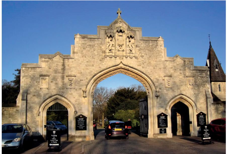
*The City of London Cemetery screen before the project: the use of impermeable cement repairs had increased the rate of decay to the point that the stonework had become unsafe. The central shield in particular was perilously close to becoming detached.*
